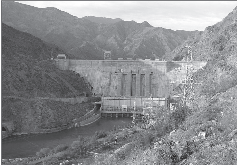
Oleg Storozhenko Kurpsai Hydroelectric Station
